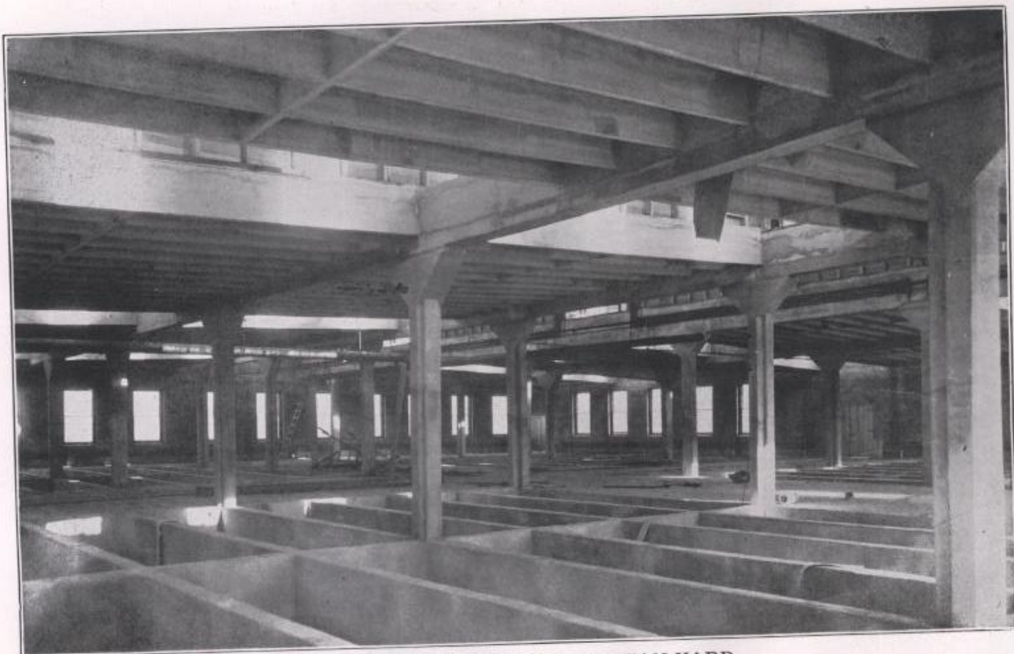
CONCRETE BEAM HOUSE AND TAN YARD. Showing Vats, Columns, Walls and Roof from the Interior of Building all constructed of Concrete.
